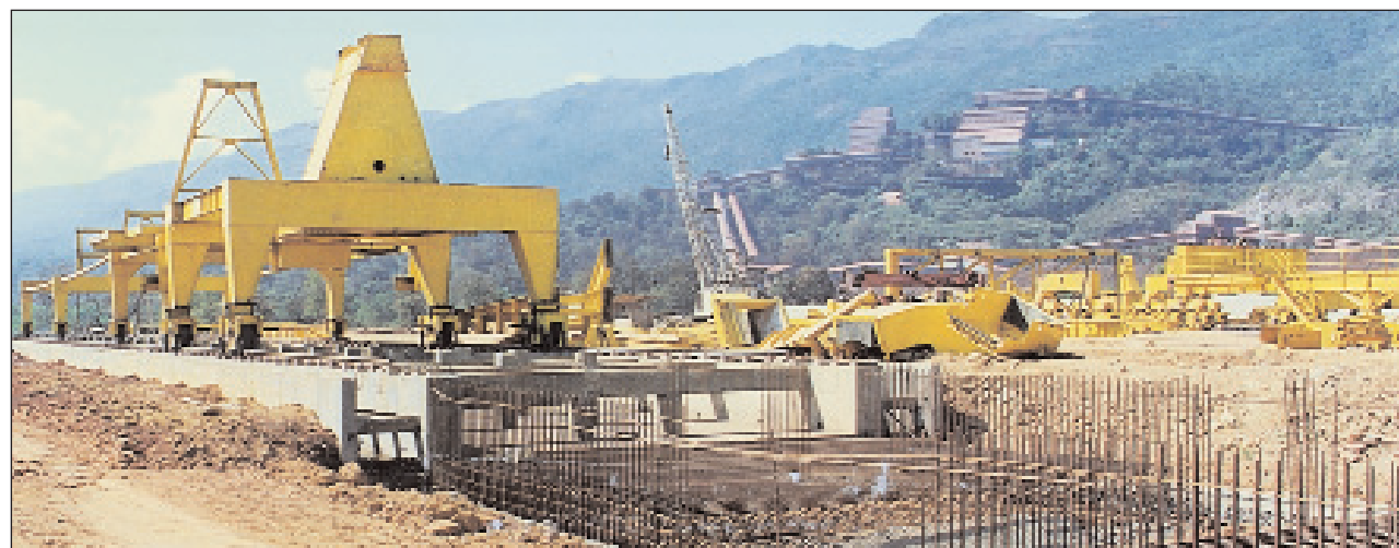
Construction work at Bailadila 10/11A Project
